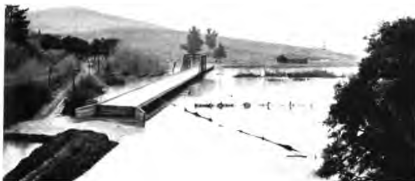
State Highway bridge near San Luis Obispo, showing flood during construction.
